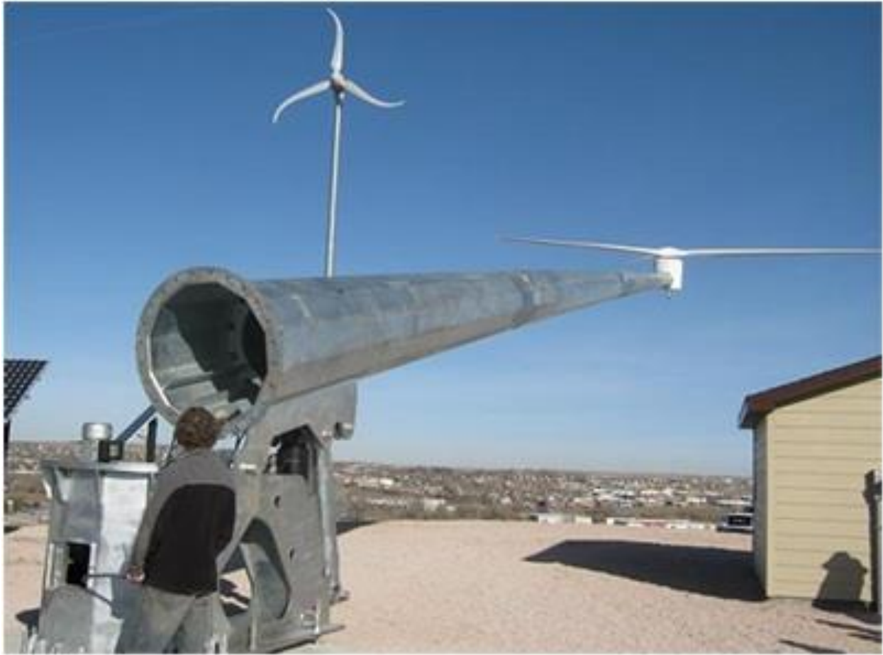
Figure 1: The hinged tower rises and lowers with a hydraulic cylinder.
