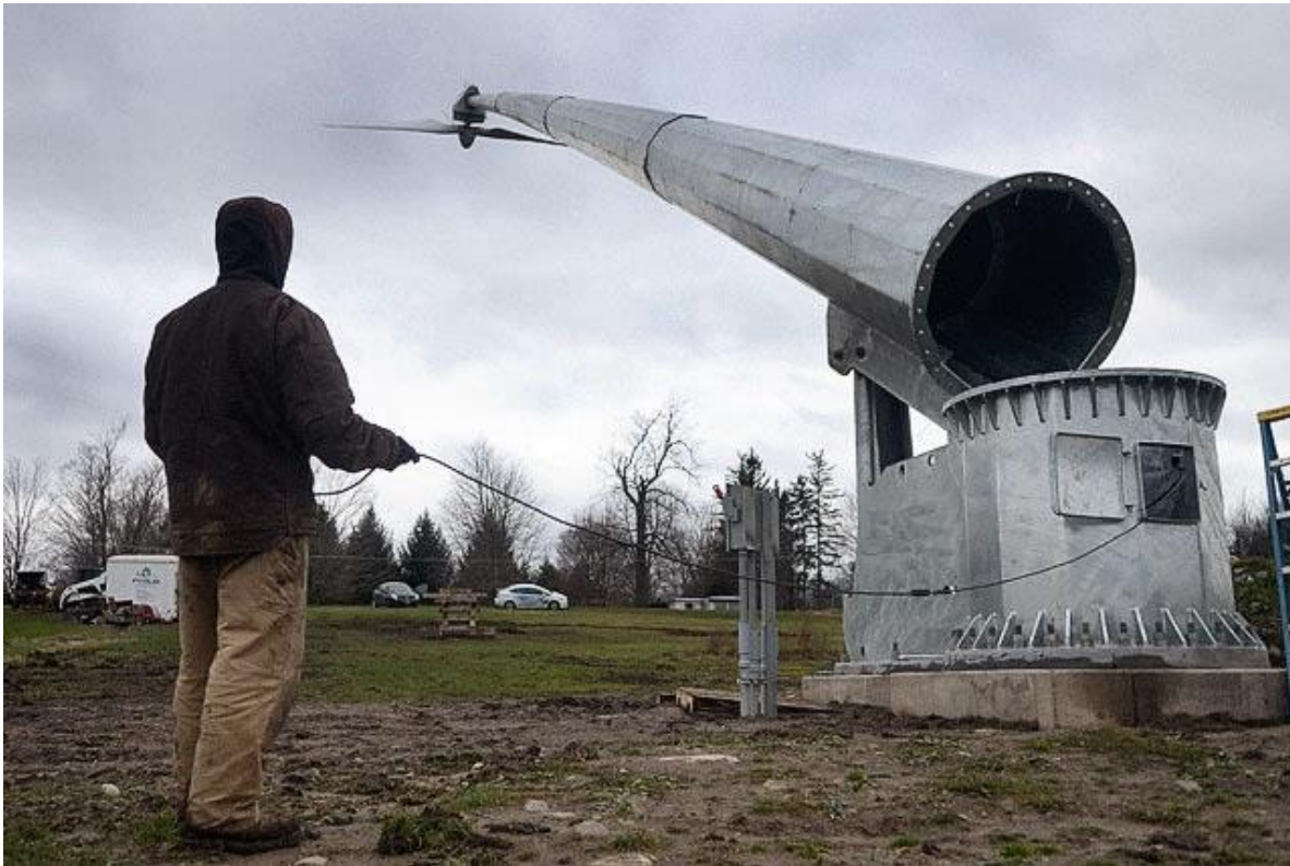
Caption: Erecting a 50 kW wind turbine tower.
